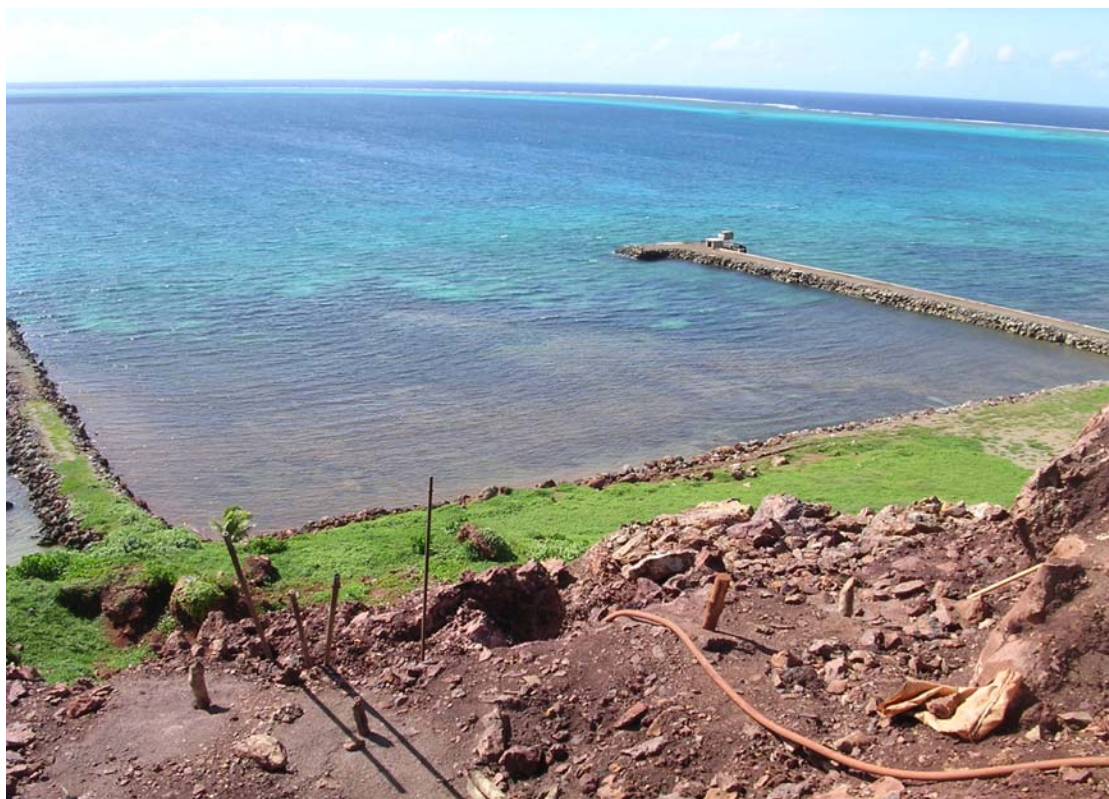
North End Runway Extension and Marina Construction
